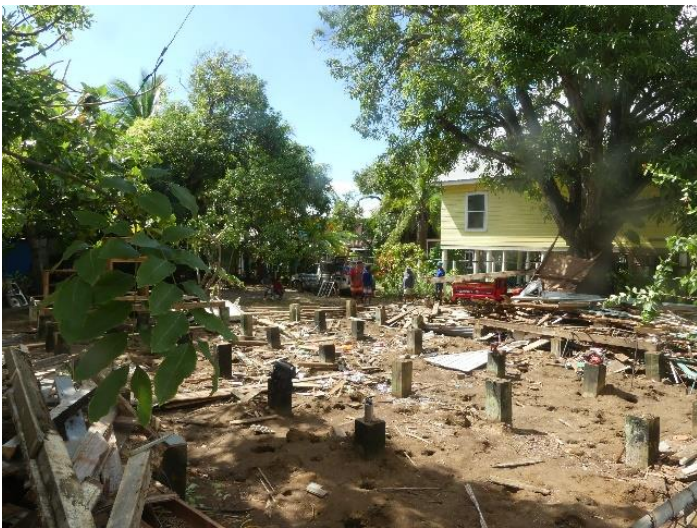
House demolition Utila style
