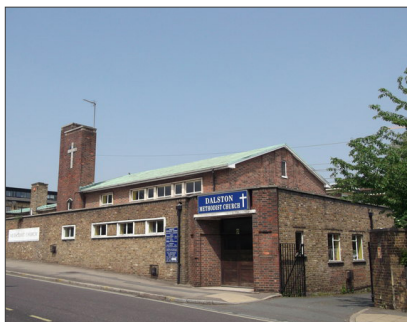
DALSTON METHODIST CHURCH MAJOR REPAIR STRATEGY ALIGNED TO CHARITIES ACT
